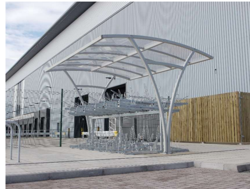
Fig 38. Secure and covered cycle shelters.
