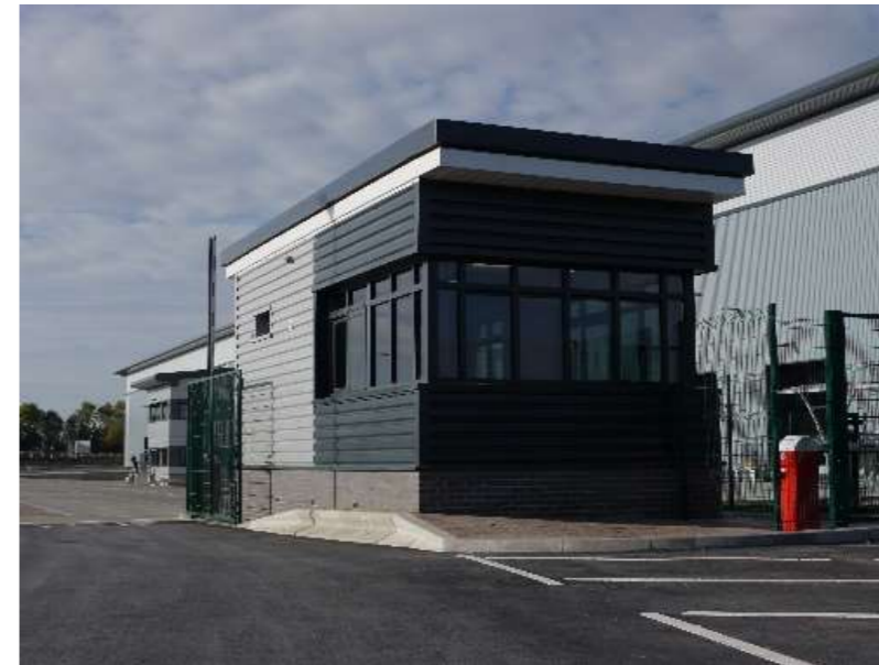
Fig 37. Gatehouse at entrance to service areas.
